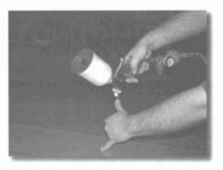
distance may vary somewhat depending upon whether you are using an HVLP system or a pressure spray gun. The spray gun should be far enough away so that the paint does not run or sag when applied, but close enough to lay on a wet coat.
