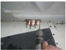
Picture 5. Drilling Door Bracket
