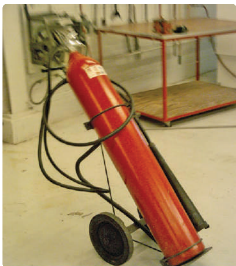
Figure 1-5. Carbon dioxide fire extinguisher.
